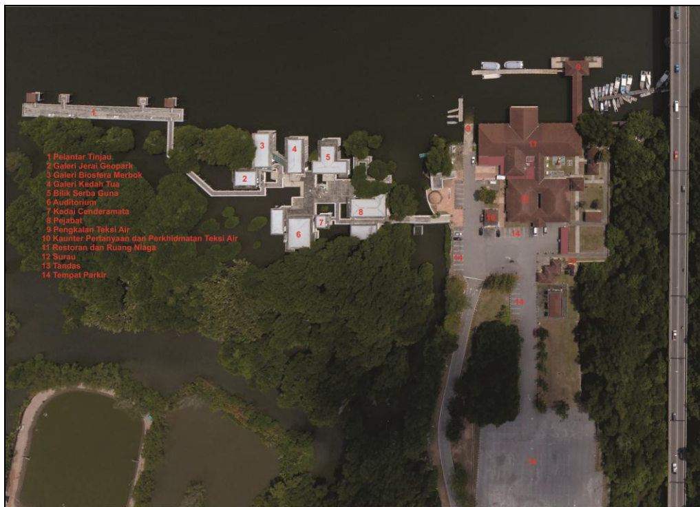
Figure 8. Kuala Muda Tourism Interpretation Center (PIPKM) which is used as a one stop center for tourism in Kuala Muda district.
